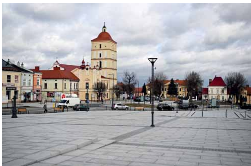
Figure 1. City square in Leżajsk: in the top photo a fragment of the square before, in the photo below the square after concreting
