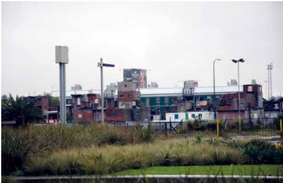
Figure 1. A view of a substandard building development at Villa 31 Buenos Aires
