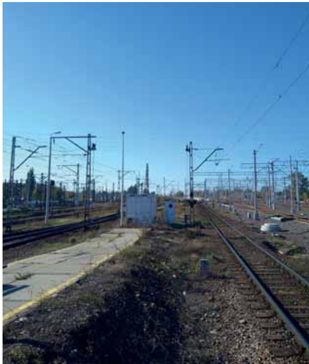
Figure 7. Railway tracks near the Warszawa Zachodnia Train Station
